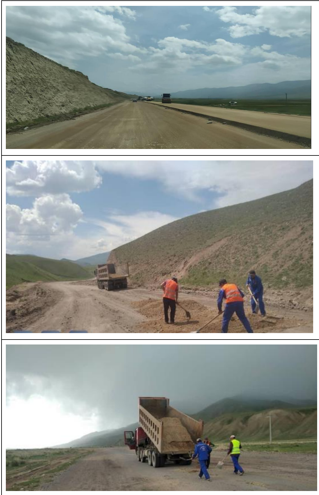
Figure 14 Road Maintenance Work
