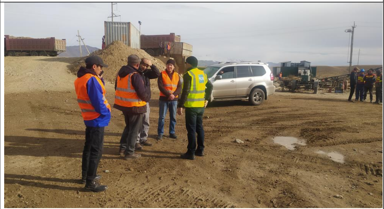
Figure 15 ADB review mission at the project site, November 2, 2022.
