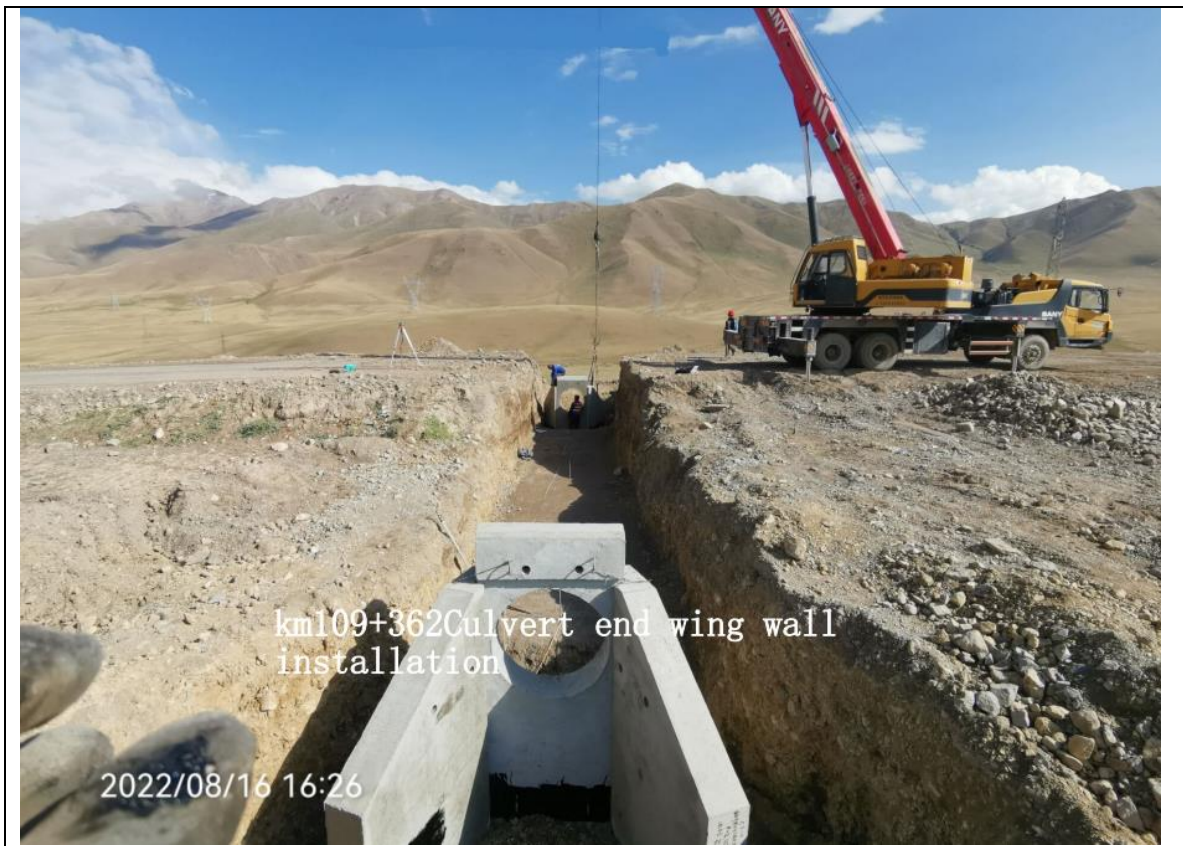
Figure 13 Constuction activities on project road.
