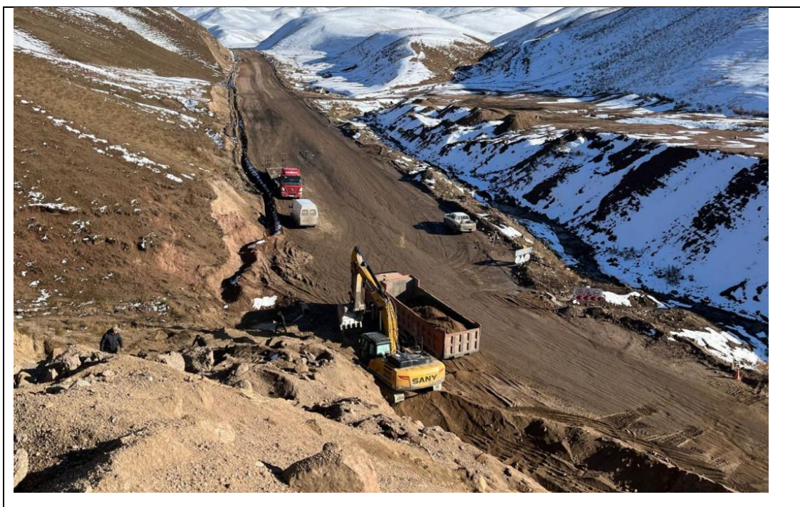
Figure 8 Road construction activities
